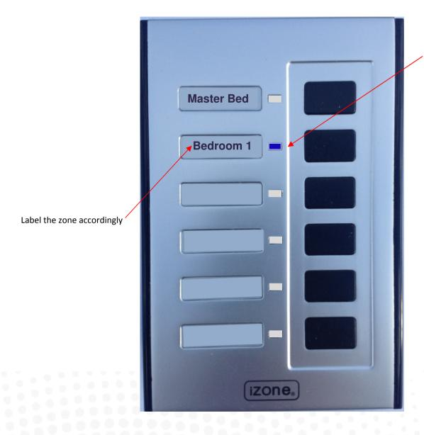
Switch all zones OFF and one zone ON. Check which zone is being supplied with air.
